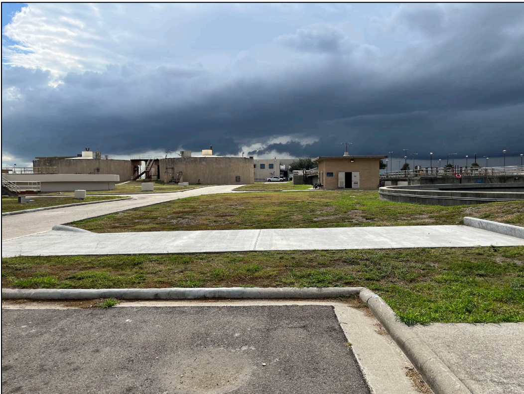
20. Photo taken from west side of WWTP facing southeast. To the left, a primary clarifier and primary digestors can be seen. To the right, a final clarifier and the dissolved air floatation thickener can be seen.
