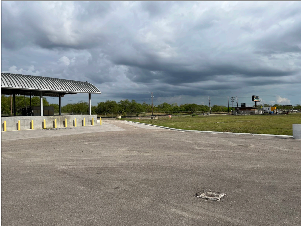
23. Photo taken from west side of WWTP facing northwest. To the left, the UV system facility can be seen. To the right, an open area, effluent pump structure, and control room are visible.
