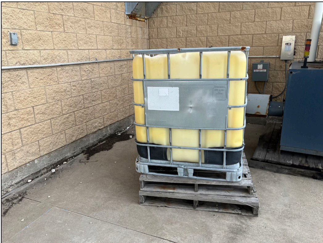
48. A container near the northeast corner of the sludge dewatering building is shown. The label was illegible.
