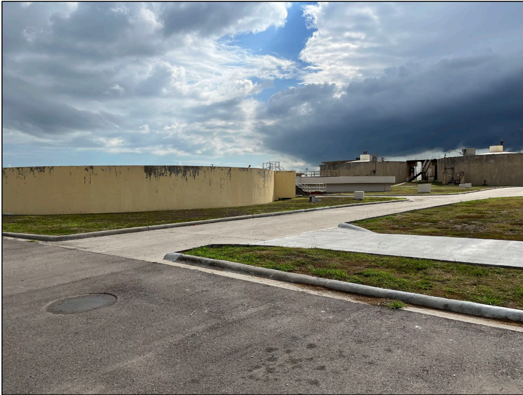
21. Photo taken from west side of WWTP facing east. Primary clarifiers and primary digesters can be seen.
