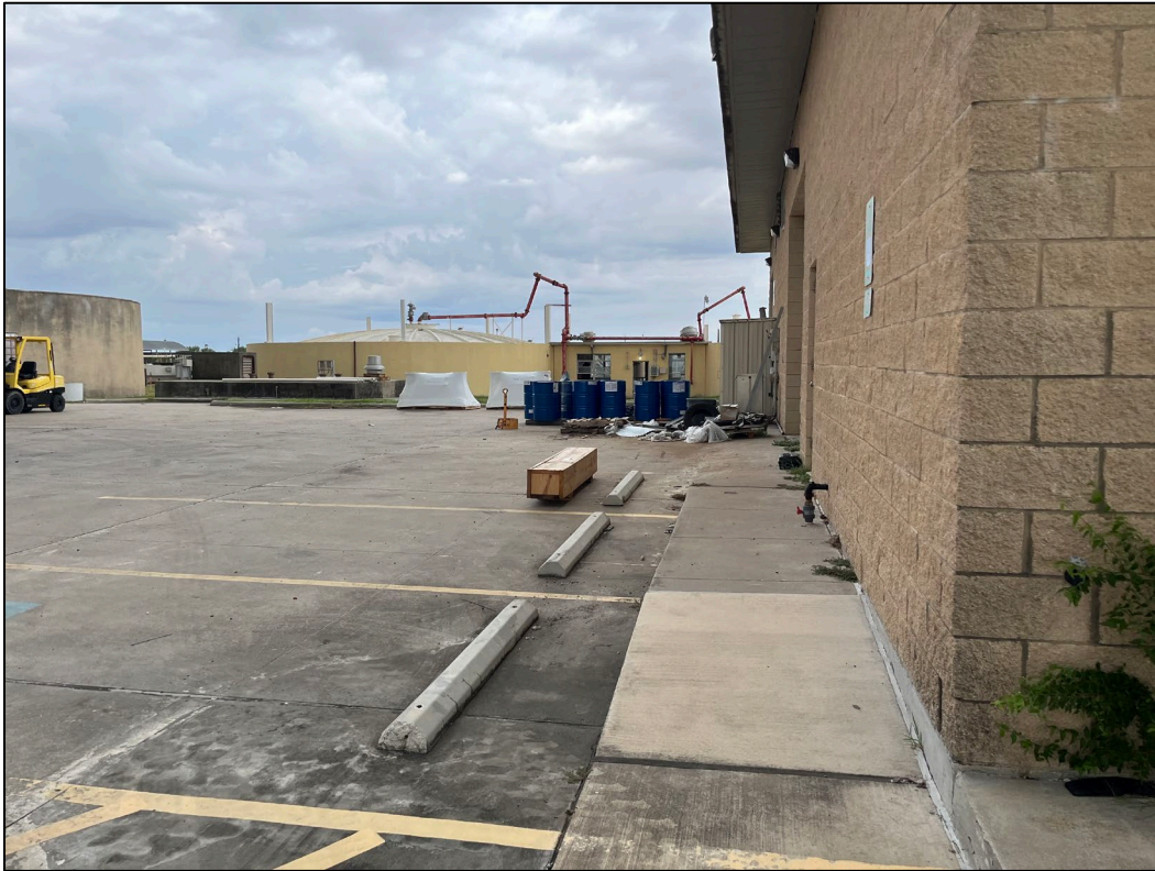
45. Photo taken from east side of WWTP facing west. To the right, the maintenance building and several drums can be seen.
