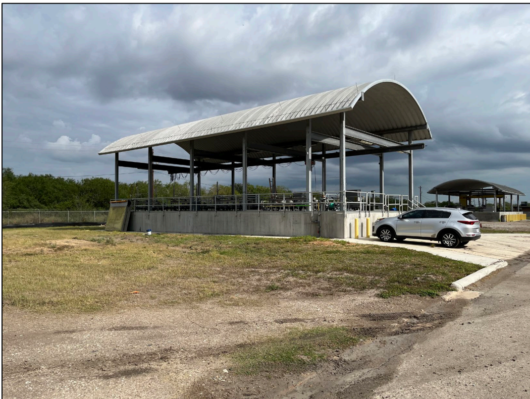
16. Photo taken on west side of WWTP facing northwest. An effluent filter system facility can be seen.
