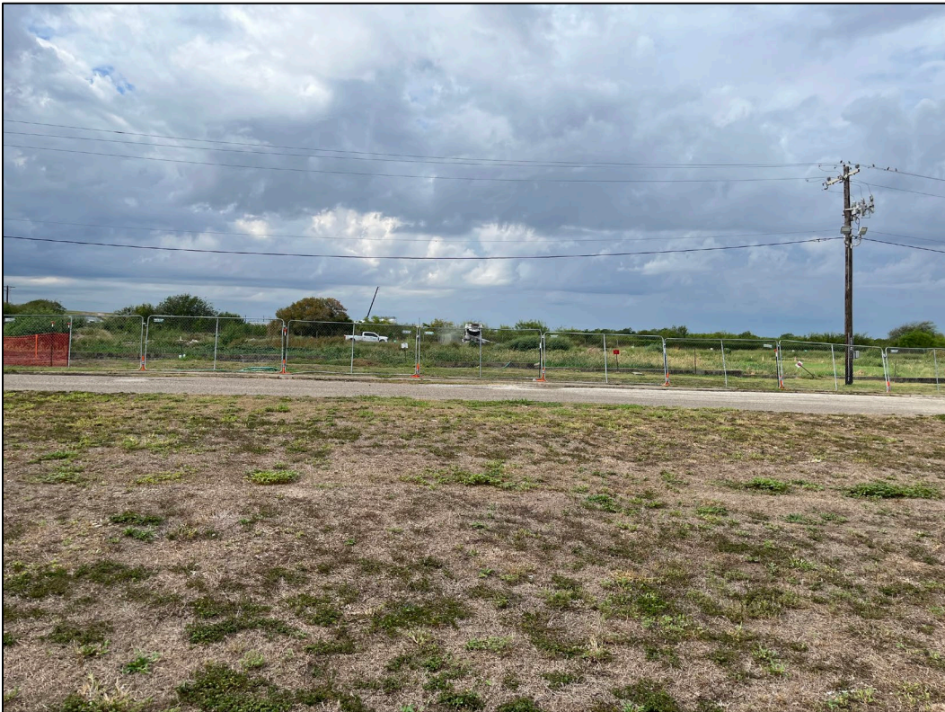
10. Photo taken on south side of WWTP facing south. Sludge drying beds can be seen on the south portion of the subject property.
