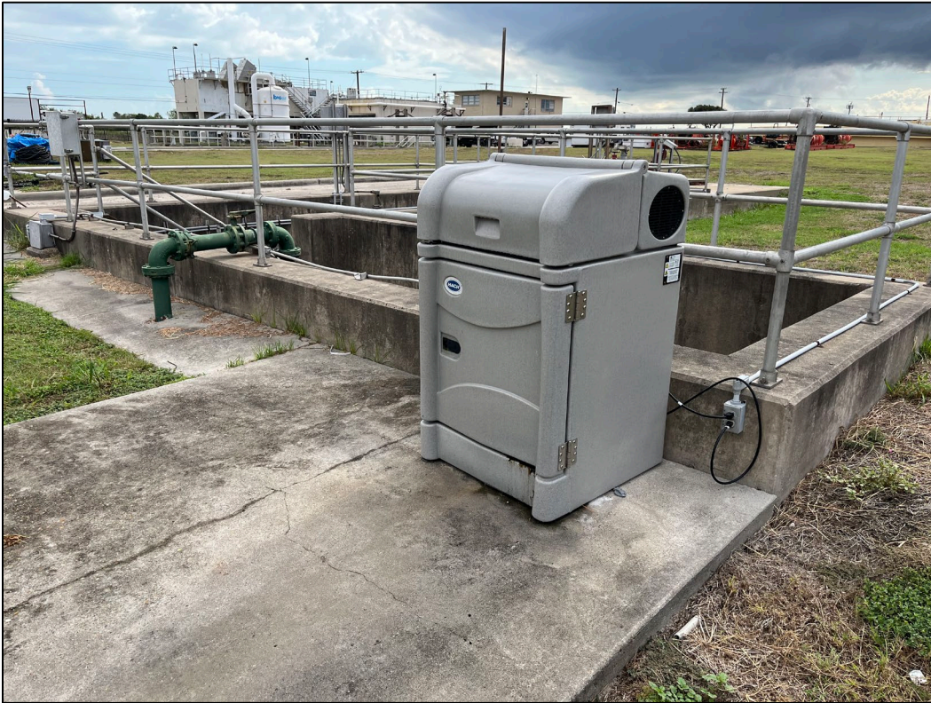
27. Photo taken from west side of WWTP facing east. An effluent sampler can be seen.
