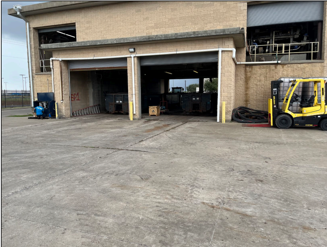
47. Photo taken from east side of WWTP facing south. The north side of the sludge dewatering building can be seen. Dumpsters for sludge storage are visible in the building. A forklift and containers of Clarifloc CE-454 can also be seen.
