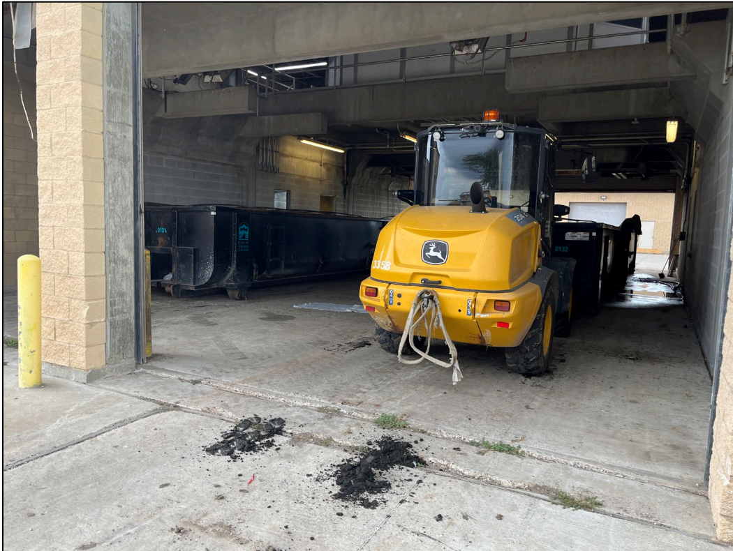
49. Photo taken from east side of WWTP facing north. The south side of the sludge dewatering building can be seen. A forklift and dumpsters for sludge storage are visible in the building.
