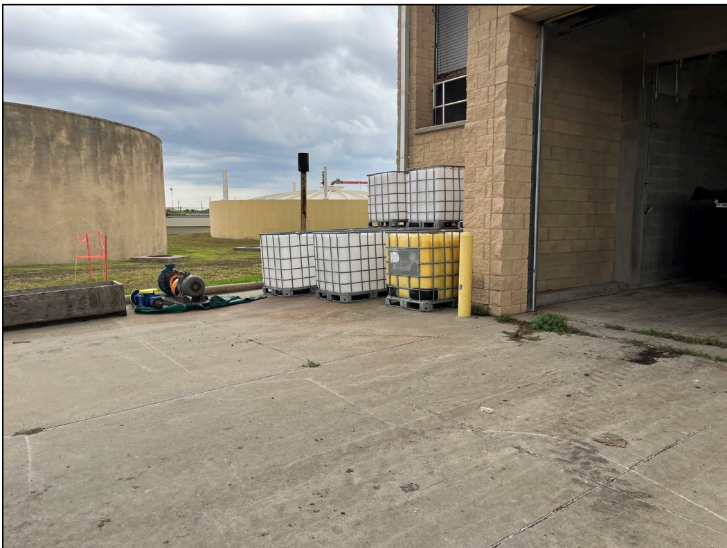
50. Containers near the southwest corner of the sludge dewatering building are shown. The containers appeared to be empty.
