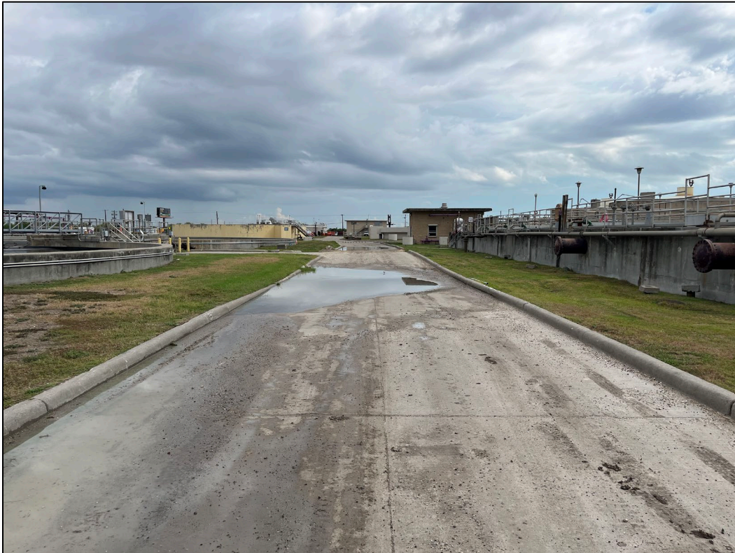
15. Photo taken in south-central portion of the subject property facing northeast. To the right of the road onsite, the aeration basins can be seen. To the left, a final clarifier is visible.
