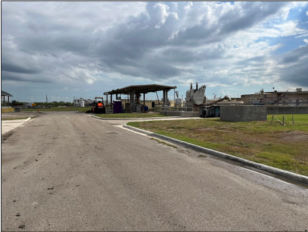
17. Photo taken on west side of WWTP facing northeast. An effluent screening facility and out-of-use UV disinfection treatment unit can be seen.
