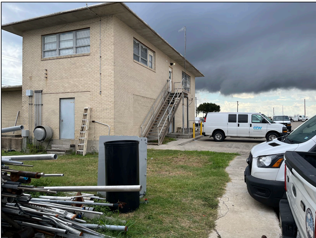
40. Photo taken in north-central portion of the WWTP facing east. An old office building can be seen.
