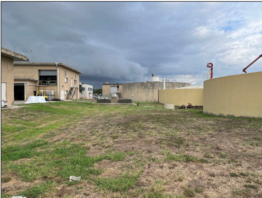
42. Photo taken in northeast portion of the WWTP facing south. Primary and secondary digesters can be seen to the right. To the left, the maintenance and sludge dewatering buildings can be seen.
