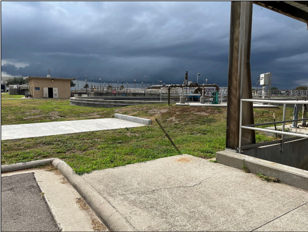
19. Photo taken on west side of WWTP facing southeast. A final clarifier and the dissolved air floatation thickener can be seen.
