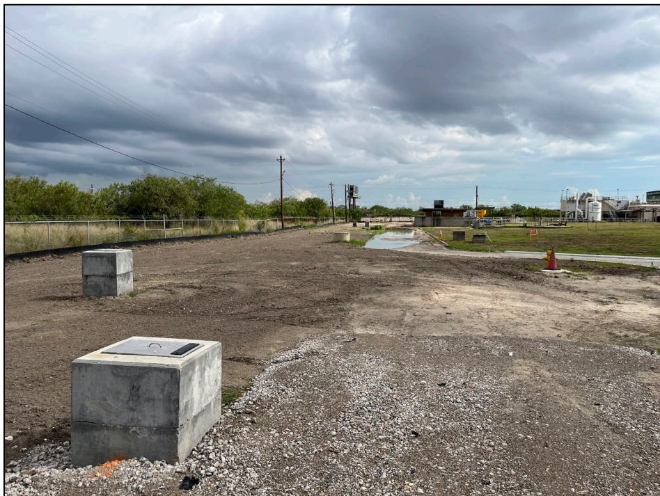
26. Photo taken from west side of WWTP facing northeast. The control room, lift station, and influent structure can be seen.
