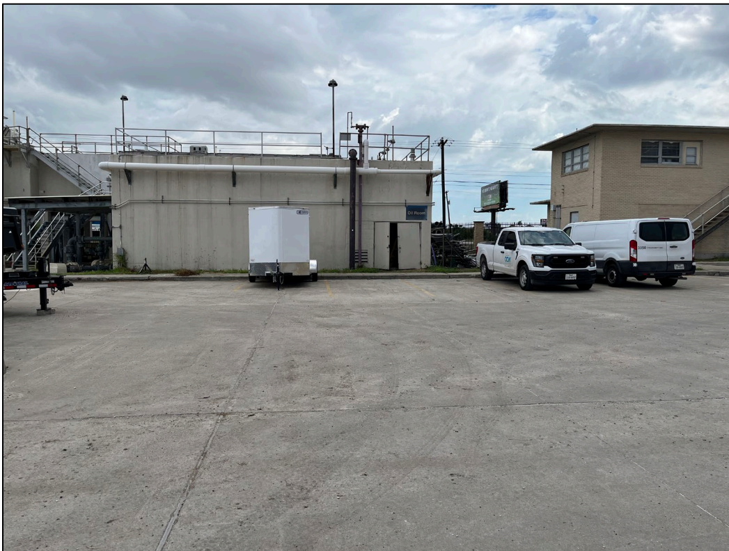
38. Photo taken in north-central portion of the WWTP facing northeast. The east end of the influent structure can be seen. The sign above the doors reads "Oil Room". To the right of the influent structure, an old office building can be seen.
