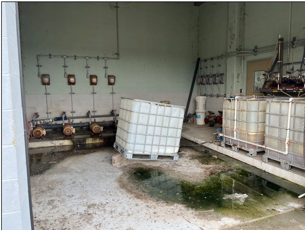
42. Photo taken near Solid Dewatering Facility in northwest portion of the subject property. Storage containers and equipment for the dewatering facility can be seen.
