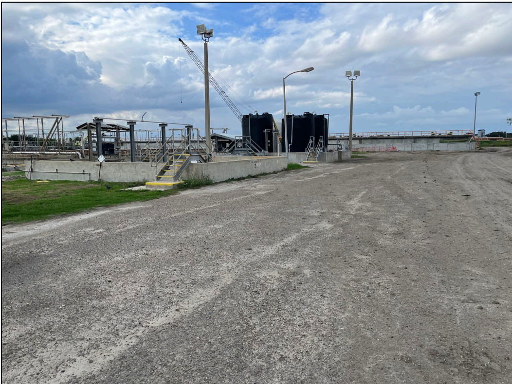
48. Photo taken from west side of subject property facing south. Sodium hydroxide and sodium hypochlorite facilities can be seen on the west side of the subject property.
