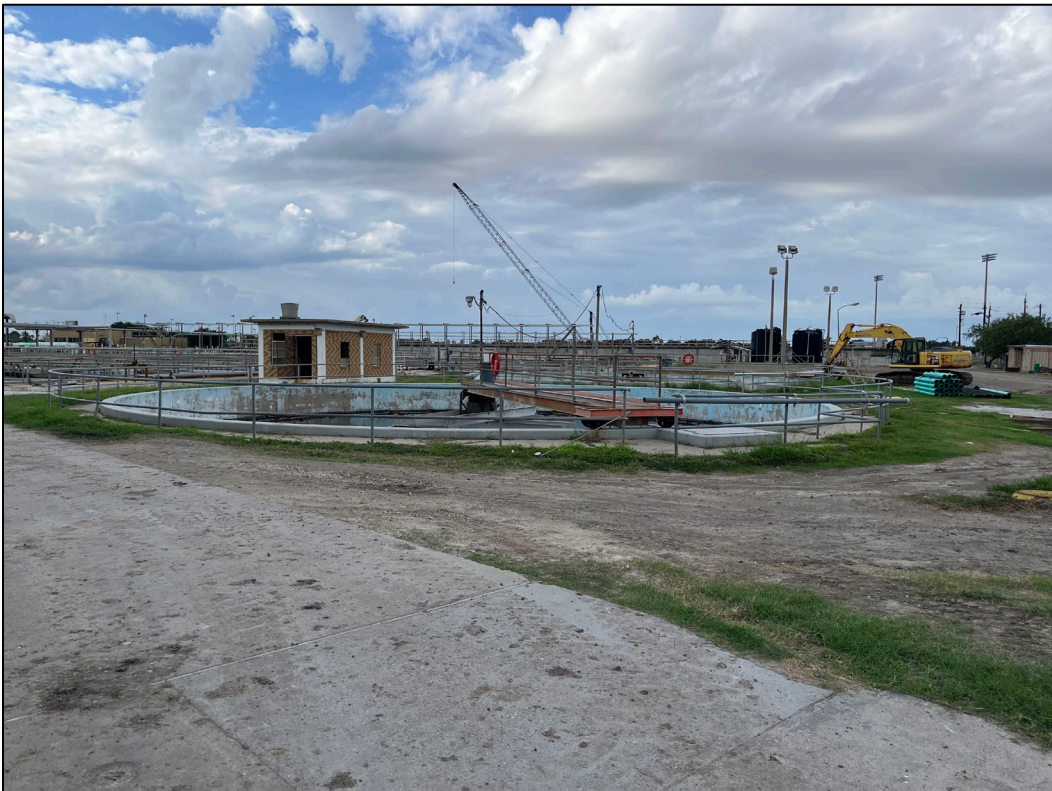
44. Photo taken in northwest portion of subject property facing south. A chlorine contact chamber on the west side of the subject property can be seen.
