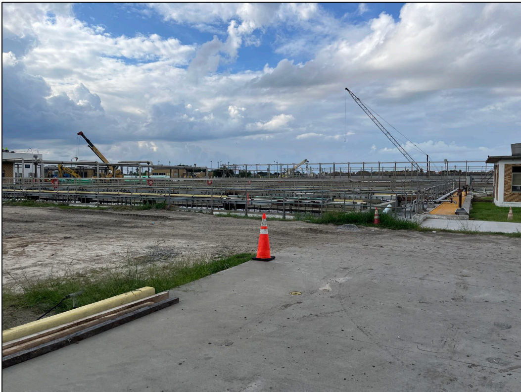
46. Photo taken in northwest portion of WWTP facing south. Reaeration tanks on the west side of the subject property can be seen. In the distance, a large crane onsite for construction can be seen.
