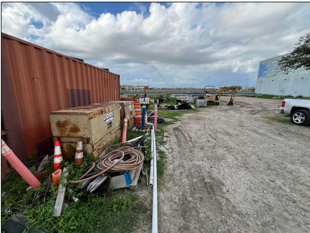
36. Photo taken in north portion of subject property facing southwest. Equipment for the construction occurring at the subject property can be seen on the ground.
