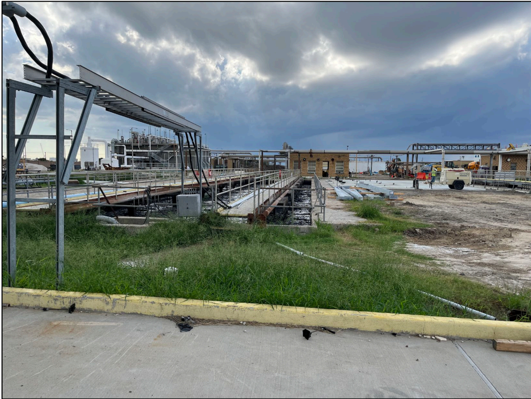
45. Photo taken in northwest portion of subject property facing southeast. An aerated sludge holding tank on the west side of the subject property can be seen.
