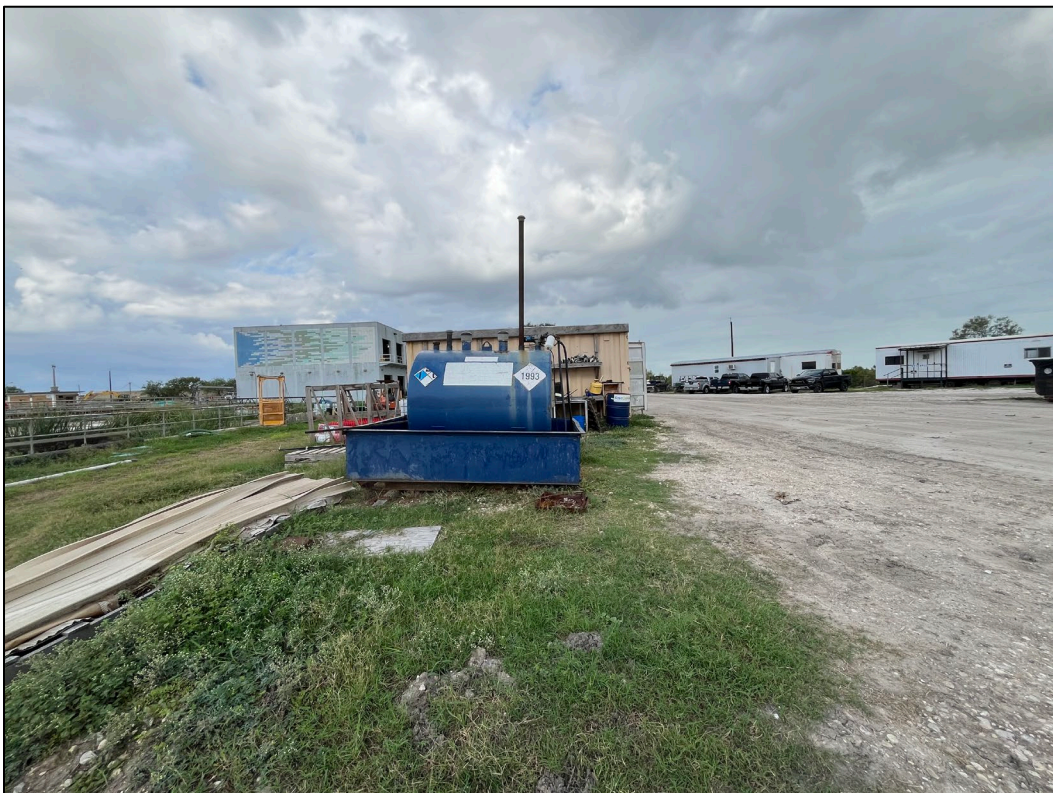
30. Photo taken west of the odor control unit on the east side of the subject property facing northwest. A diesel aboveground storage tank with secondary containment and storage containers can be seen.
