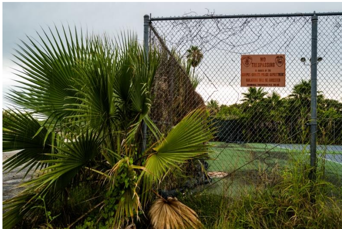
Figure 10 Former tennis facility of Pharoah Valley Golf Course
